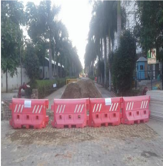
Provide Proper Barricading and Signage for Excavation Work and Maintenance Work
